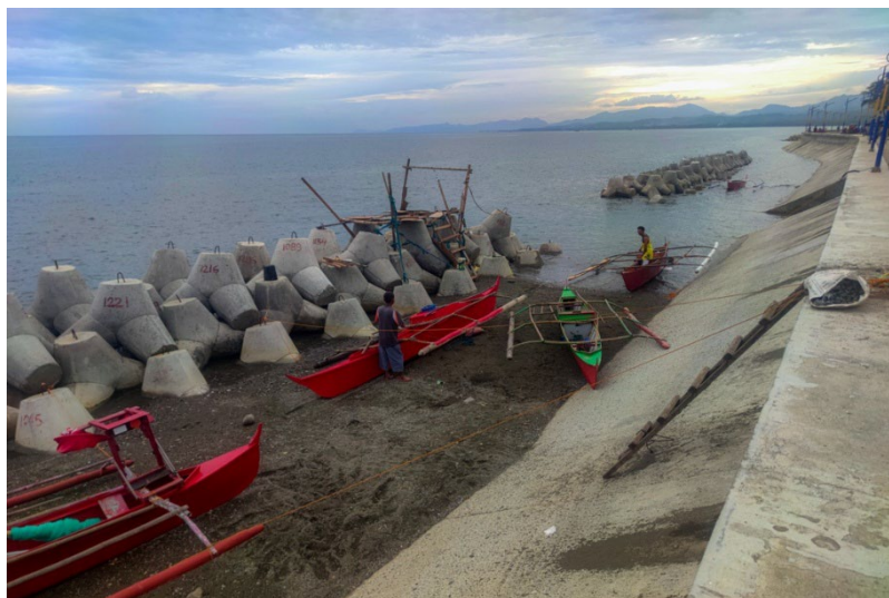
Figure 4: Concrete-based seawall on the right with artificial wave-breakers on the left. This allows limited docking places for the SSF. (Quitag, 2025)
